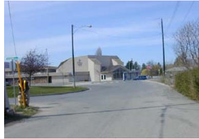
Larch Avenue, looking west past Kitchener Drive to Fortune Drive. The presence of a channelized right turn shortens the weaving distance.
