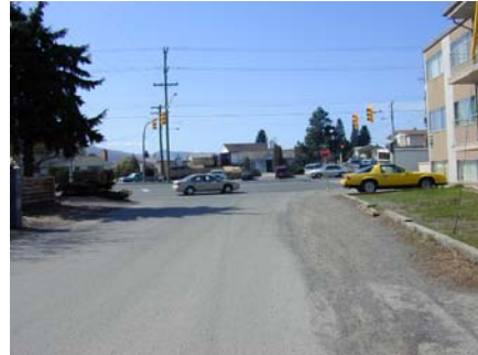
At the east leg at Oak Rd. and Fortune Dr. the driveways and parking are very close to the intersection.
