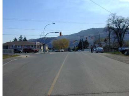
Lack of delineation on channelized right-turn lane, combined with a driveway on the exit leg may lead to conflicts
